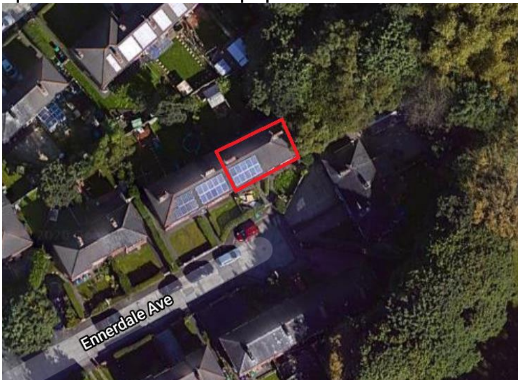
Aerial view of the two properties to be demolished
