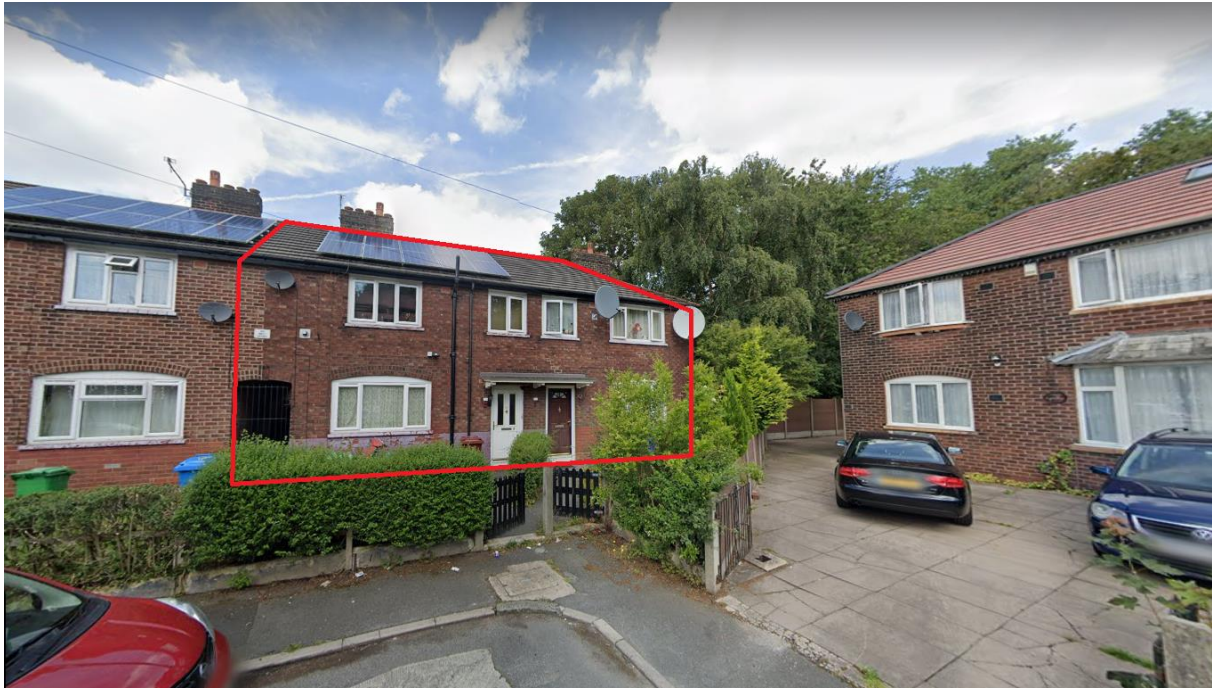
The two properties to be demolished in order to extend Ennerdale Avenue and develop the land to the rear of these properties.
