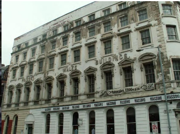
2006 Prior to erection of Scaffolding
