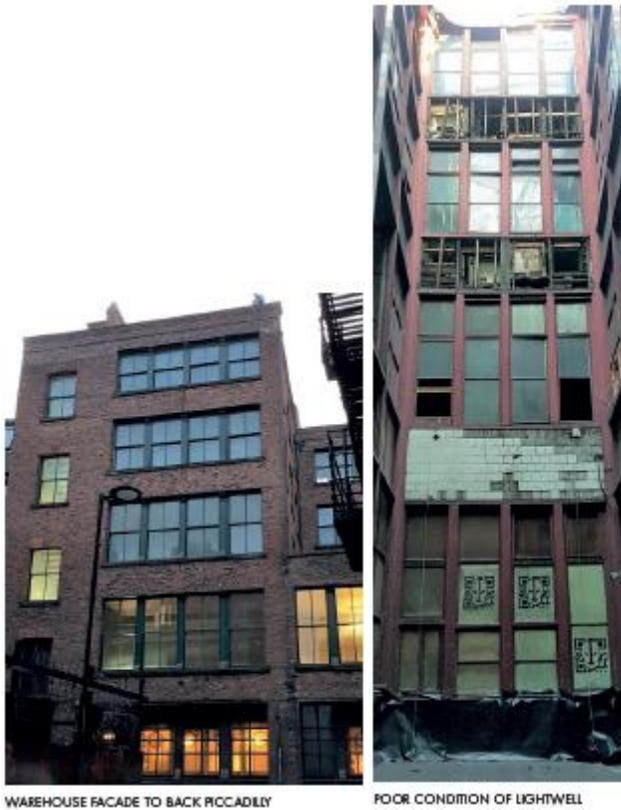
WAREHOUSE FACADE TO BACK PICCADILLY
